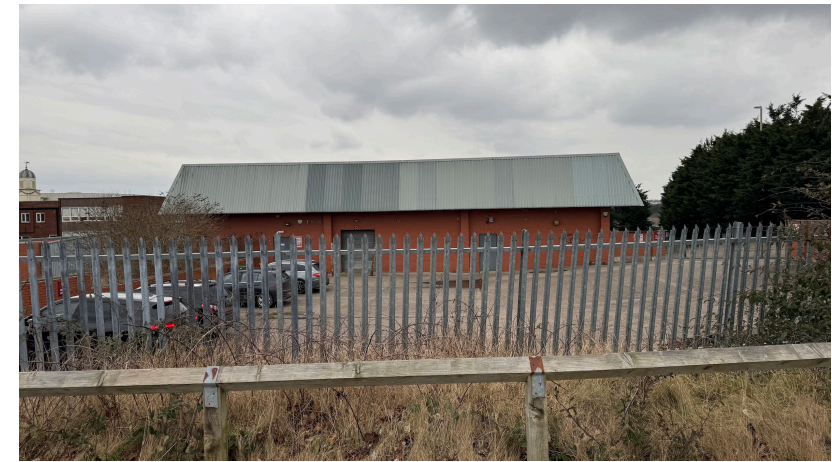
2. View of the first Floor Loading bay elevation from The East.
