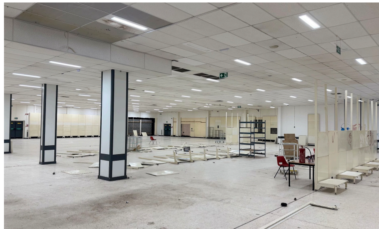
5. Interior view of existing ground floor retail space
