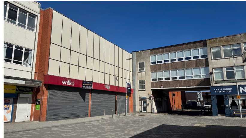
9. Ground Floor Retail Entrance to Market Place
