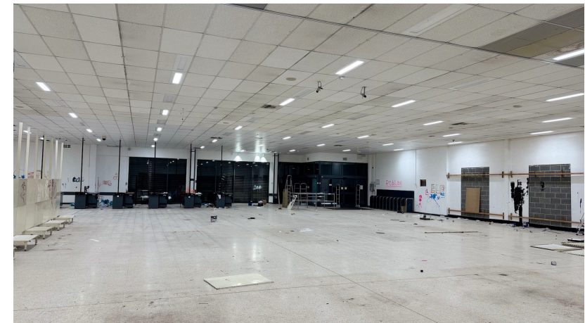
6. Interior view of existing ground floor retail space
