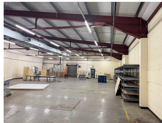
11. Interior view of Existing First Floor Warehouse.
